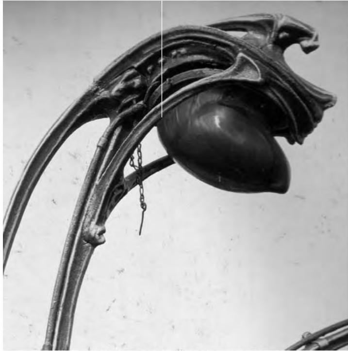
Figure 27 Stalk on type A station containing lamp
