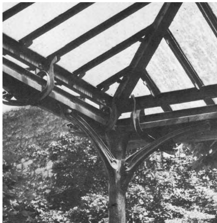
Figure 32 Column-roof detail inside Porte Dauphine station
