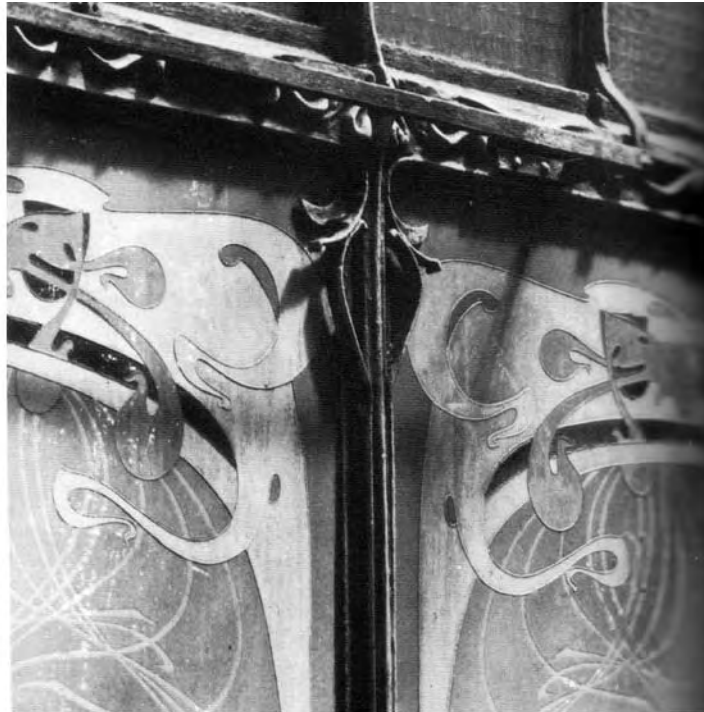
Figure 31 Iron and stonework detail inside Porte Dauphine station
